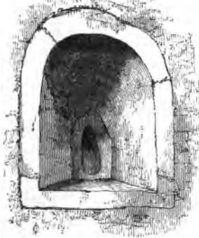
10. Window with small opening and very wide splay, Caversfield, Buckinghamshire
